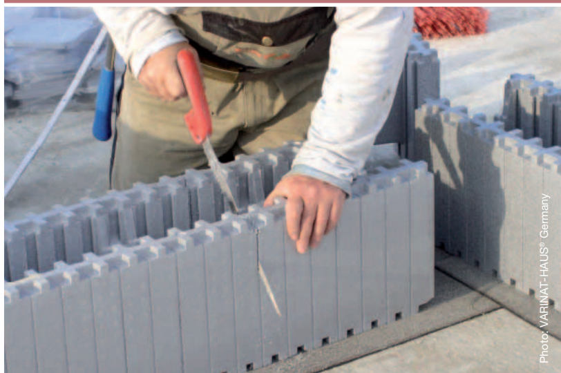
Precise and fast cutting to size with a handsaw
